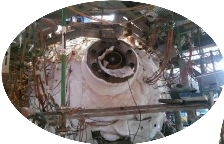
Repair of HP Scrubber sphere
