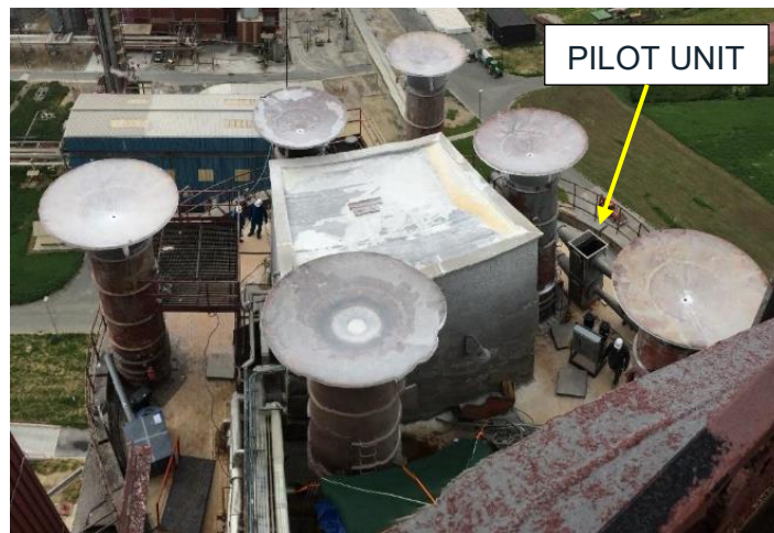
Figure 5: In-field pilot testing.
