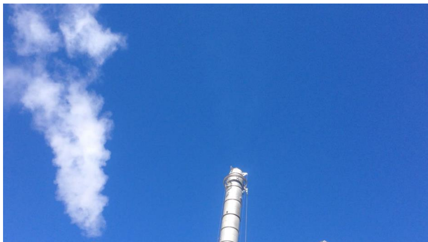
Figure 6: Zero opacity observed at the stack outlet (photograph taken at one of the reference plants).
